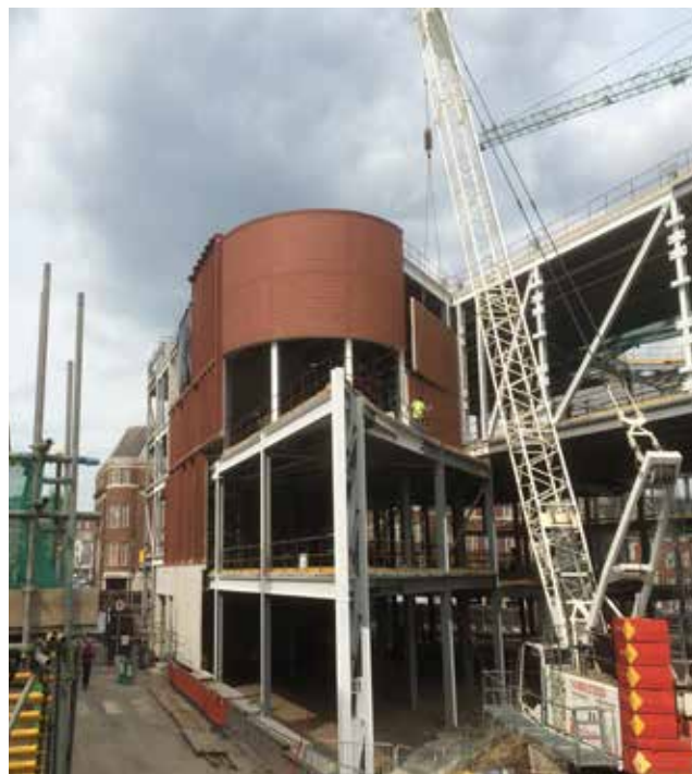
ACME Victoria Gate Arcade, Leeds.
